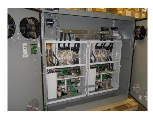
Induced Draft Fan Inverters for Boiler Control. Example 400 HP. Customer: Clarage, USAF base, Eielson, Alaska
