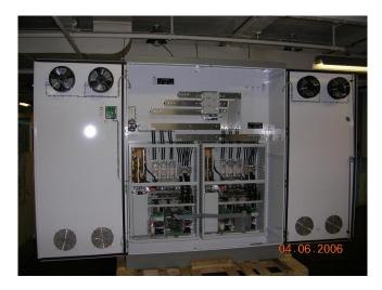
• Autoclave Inverters for the Military and Commercial Aircraft Industry. Example: 300 HP. Customer: Taricco
